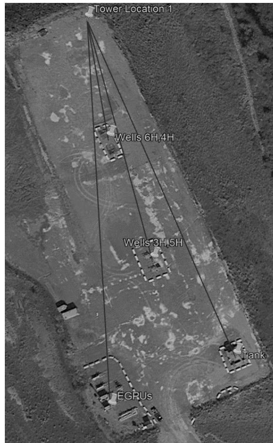
Figure 5.1: Initial location of the eddy covariance trailer tower with respect to major components at MIP (MSEEL 1.0).
