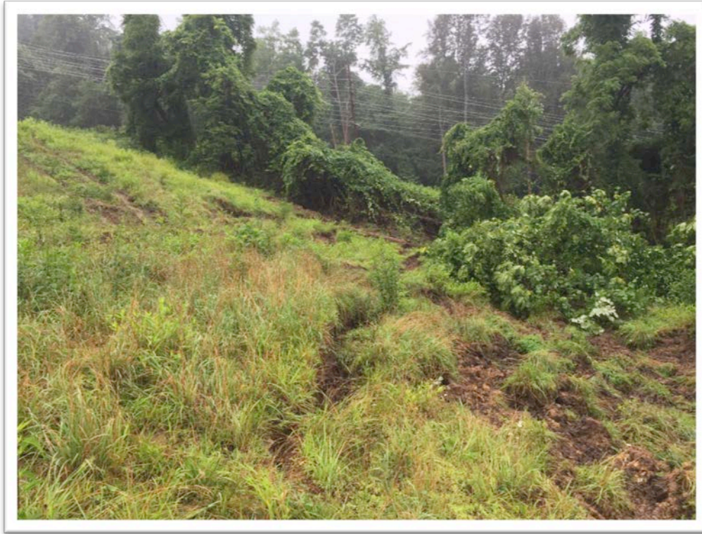
Figure 2. Landslide mass above WIP Science Pad
